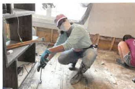
Removing damaged flooring was one way the students assisted homeowners.
